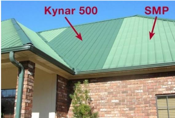
Both Kynar and SMP panels were the same color when installed on this project. The picture was taken 8 years later - Kynar looks the same as the day it was installed while SMP is showing significant color fading and chalking.
